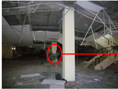
Photo 10 Damage of Inside Columns of the Building
