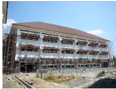
Photo 1 College under Construction (UMY)
