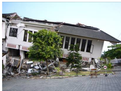
(b) Story-Collapsed Building
