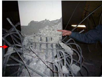
Photo 10 Damage of Inside Columns of the Building
