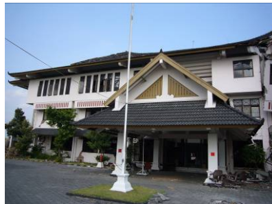
(a) Slight Damaged Building
