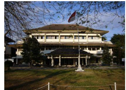
(a) Slight Damaged Building
