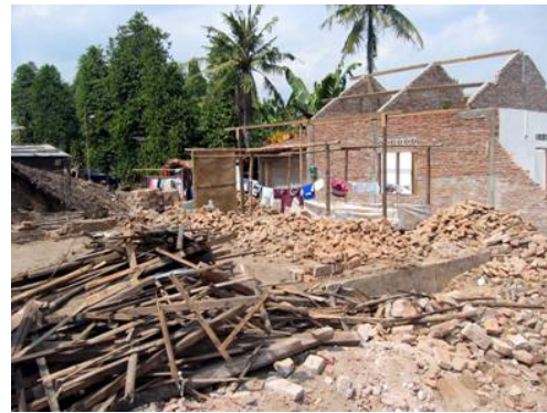
Photo 15 Damage to Residences
