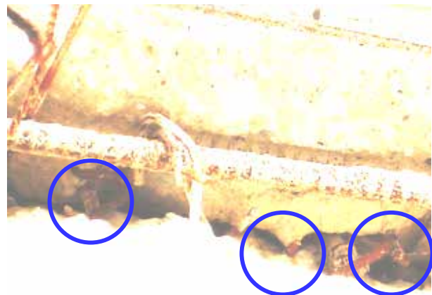
Figure 13. Zoom viewing of wall anchor
