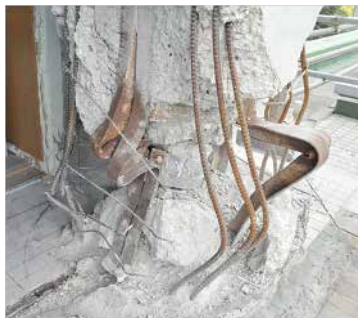
Figure 11. X8-Y2 column after remove the crush concrete
