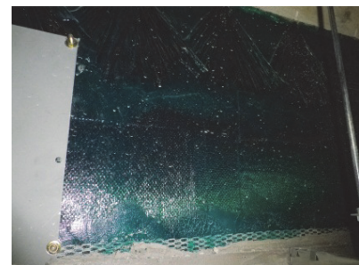
Photo 4 Stuck carbon fiber reinforcement with anchors
