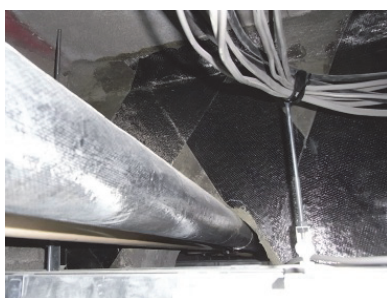
Photo 2 Stuck tape-shaped carbon fiber
