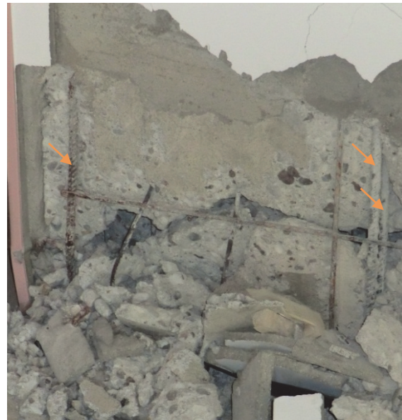
Photo 14 Detail of bars from the other side of photo 13
