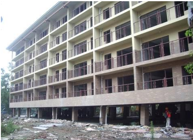
Photo 10 Example six story RC partment building (See also Photos 6 and 7)
