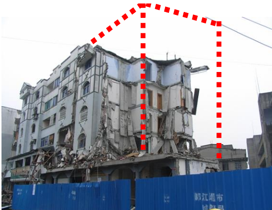
Photo 1 Seriously Damaged Brick Buildings (Hanwang town of Mianzhu city)
