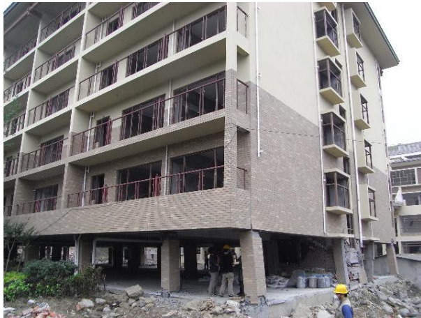
Photo 6 General view of a six story RC apartment house
