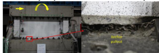
Fig. 6 Overall flexural failure as observed in [10]
