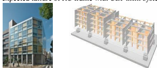
Fig. 1 Examples of steel frame with CLT infill (left) [4], RC frame with CLT infill (right) [5] buildings
